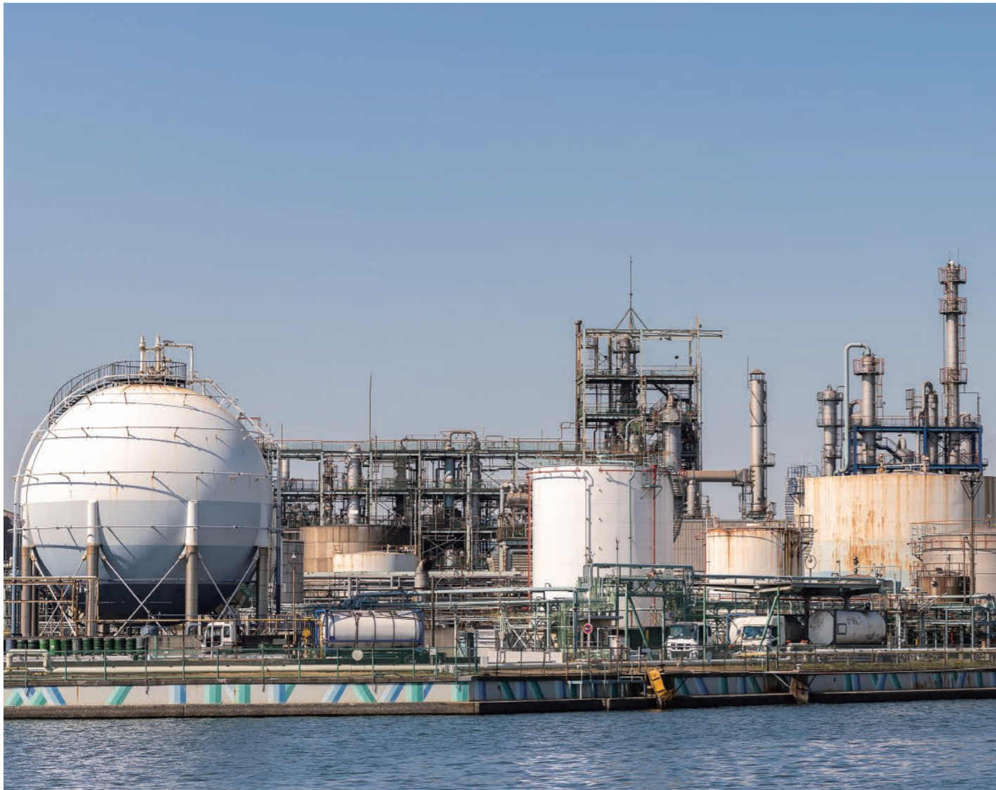
SPON's IP HD Surveillance Microphone System, tailored for unique industry needs with specialized technology and experience, is widely used in industrial, chemical, mining, and correctional facilities.
