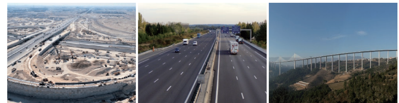
Al Khor Expressway (Qatar)
