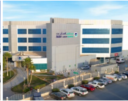
Aster Sanad Hospital Riyadh (Saudi Arabia)
